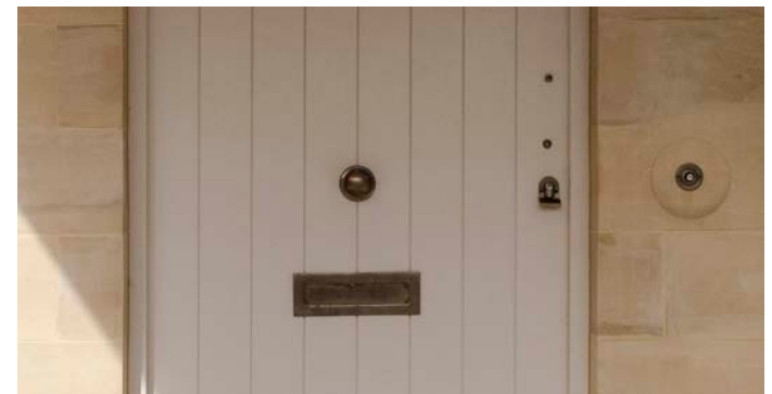
Bell Push integrated into stonework feature, rather than an afterthought.
